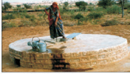
Recessed Tanks टाँका
